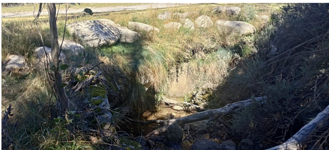
Figure 15: Watercourse/head wall of piped section below road surface
